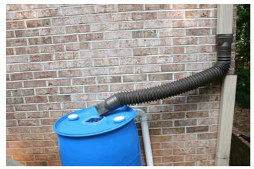
8. Glue 2"PVC fittings and pipe as needed to direct overflow water away from your home's foundation. When the barrel is full (or when you do not need to store water), you can slip the 16" piece of downspout into place on your home gutter downspout to direct water through it and away from the house.
