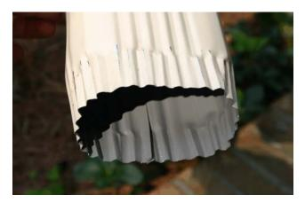
6. Cut an opening into the other end of the 16" piece of downspout as shown here.
