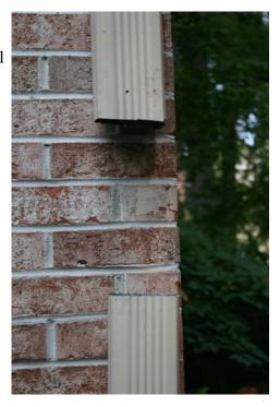
5. Cut a 16" piece of downspout from the new piece you purchased. One end should be crimped as shown.
